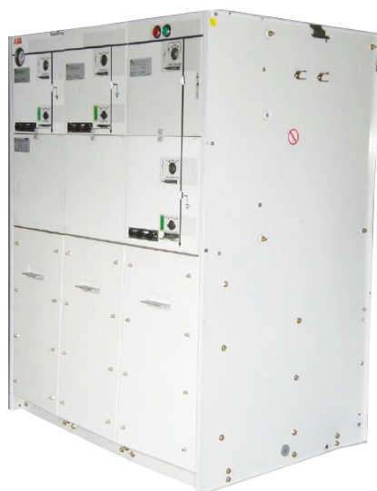
From IAC-test with arc suppressor
